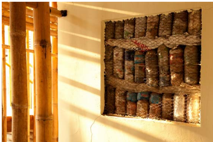
Photo 23. Detail of the construction of the wall KoukKhleang Youth Center
